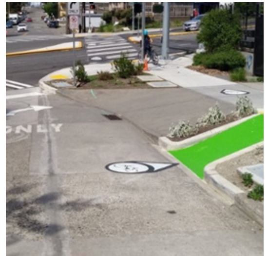
Figure 70: Example of a bike wayfinding dots used to guide users through an intersection
