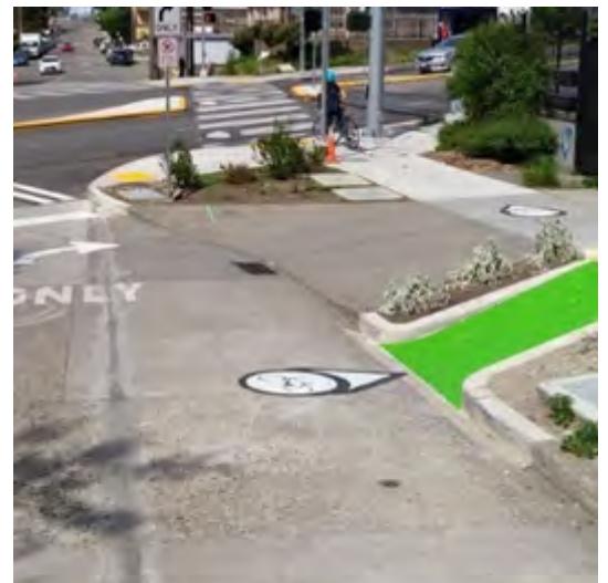
Figure 70: Example of a bike wayfinding dots used to guide users through an intersection
