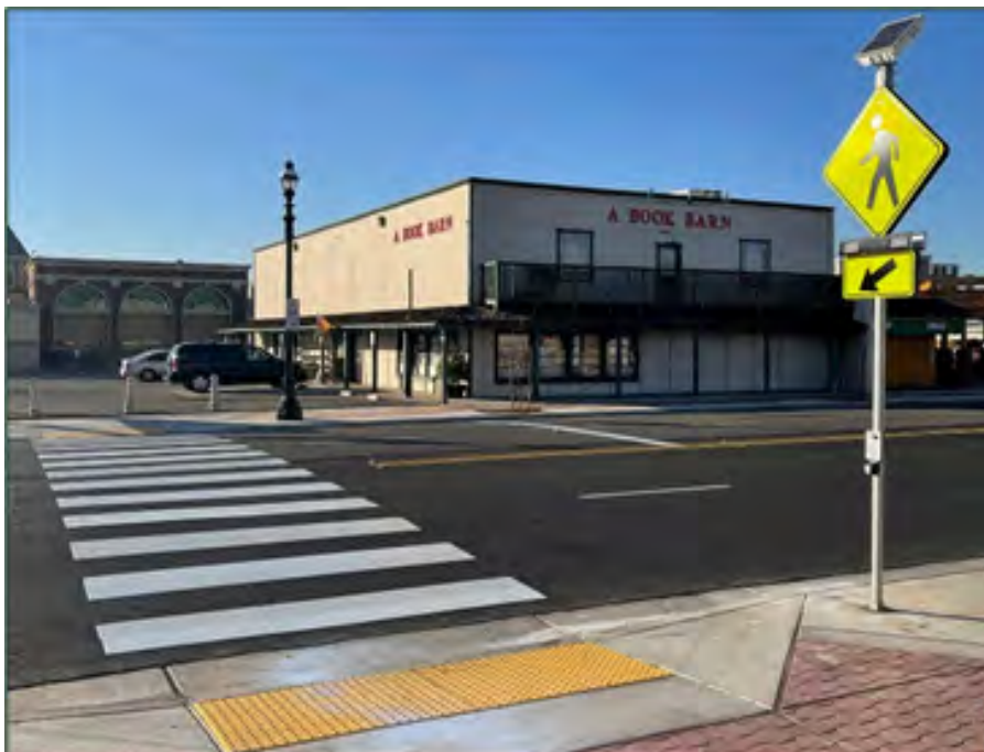
Figure 27: Rectangular Rapid Flashing Beacon (RRFB)
