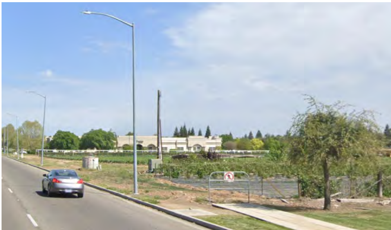
Figure 4: There is a Gap in the Sidewalk Network on the South Side of East Herndon Avenue between North Willow Avenue and North Peach Avenue
